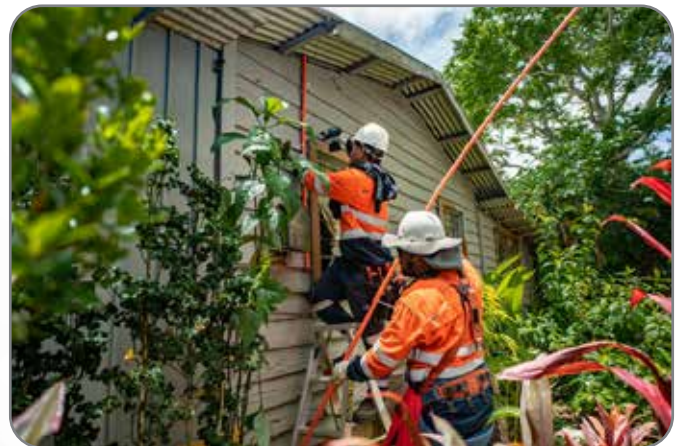
Installation of electric conduits on building walls
