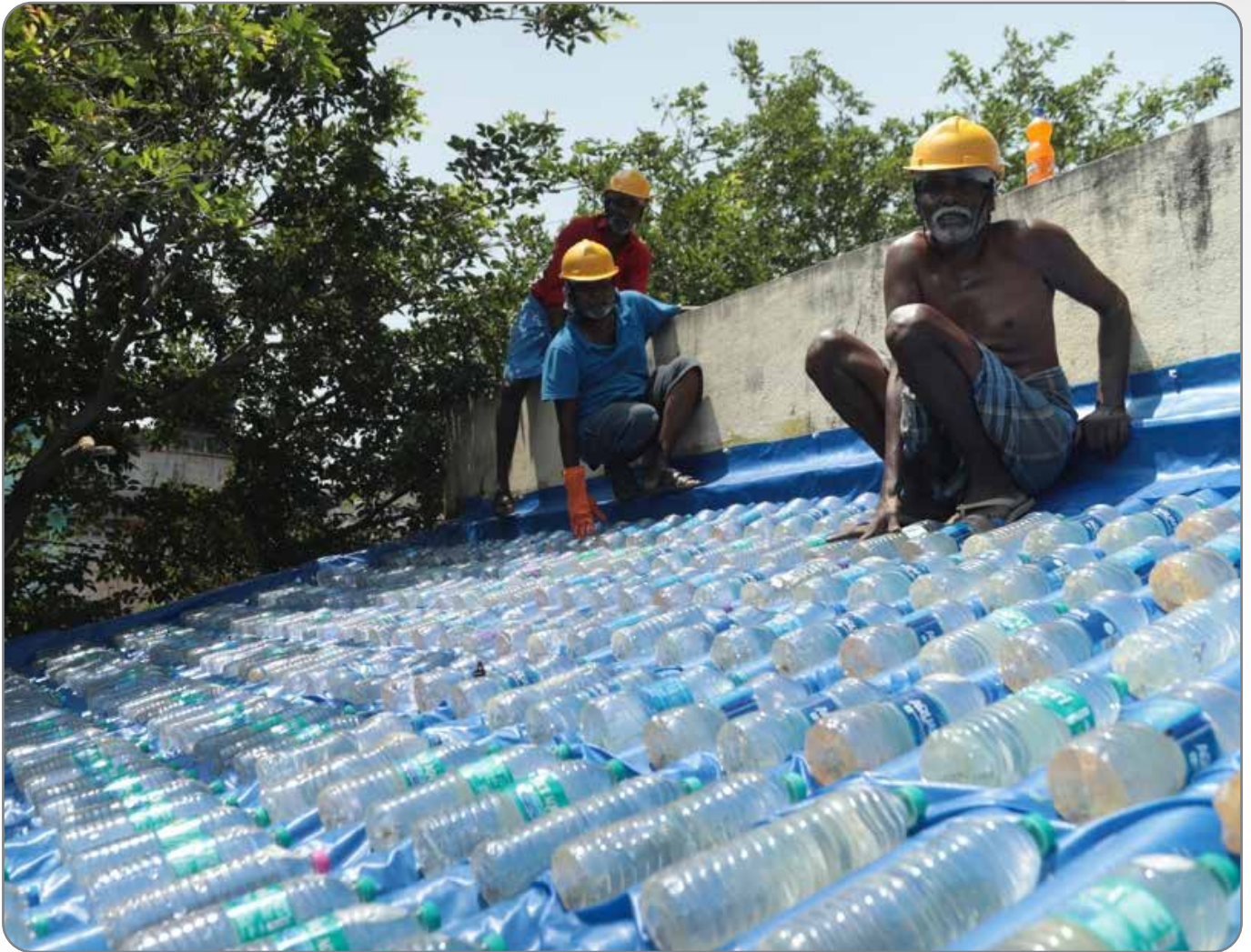
Installation of PET Bottles on a community centre in Chennai, India.
