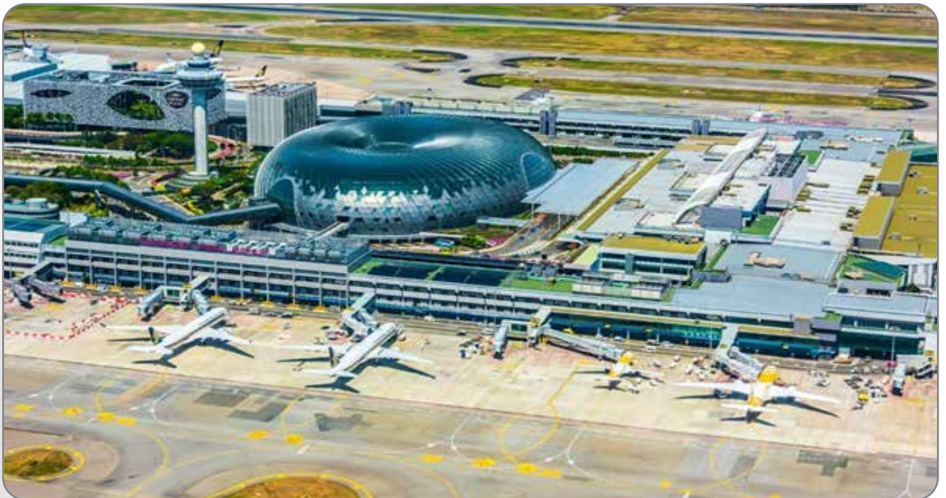
Changi Airport Source: Royal HaskoningDHV
