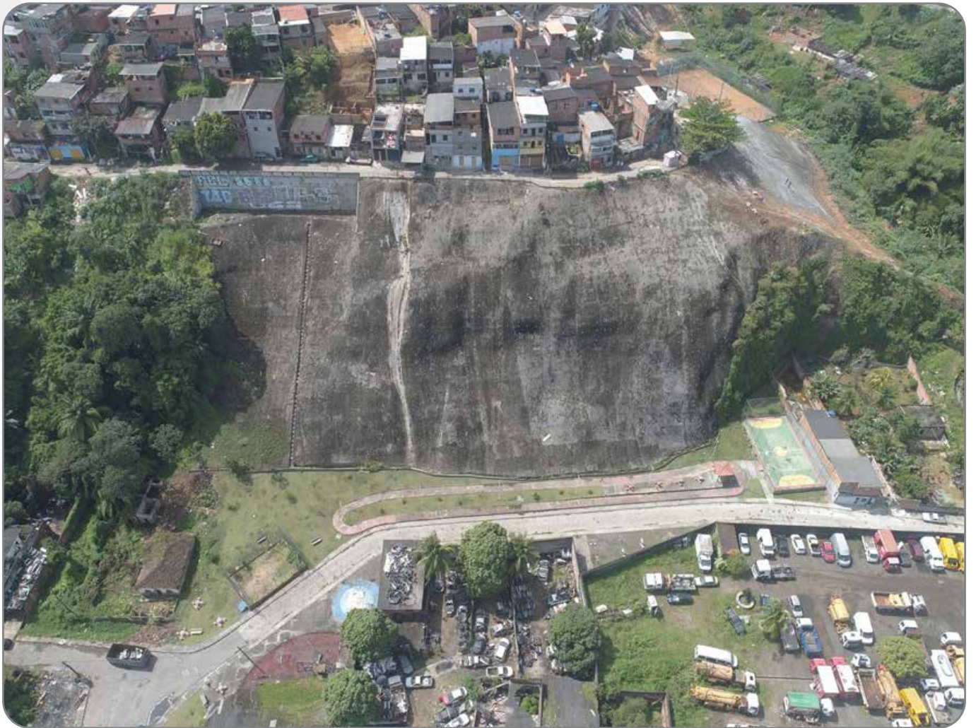
Slope Containment and Slum Urbanization at PDE 124
