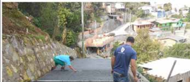
Paving in Caiera Community
