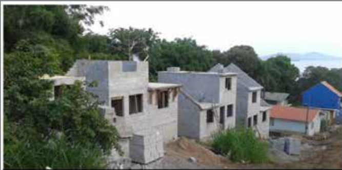
Structural Masonry House at Nova Descoberta Community
