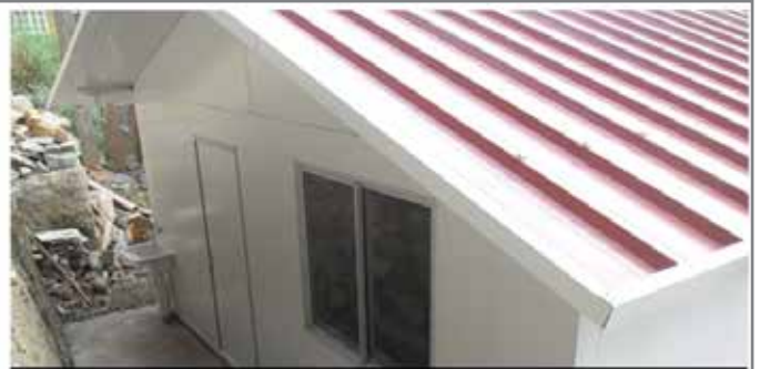
Modular House at Morro do Céu Community
