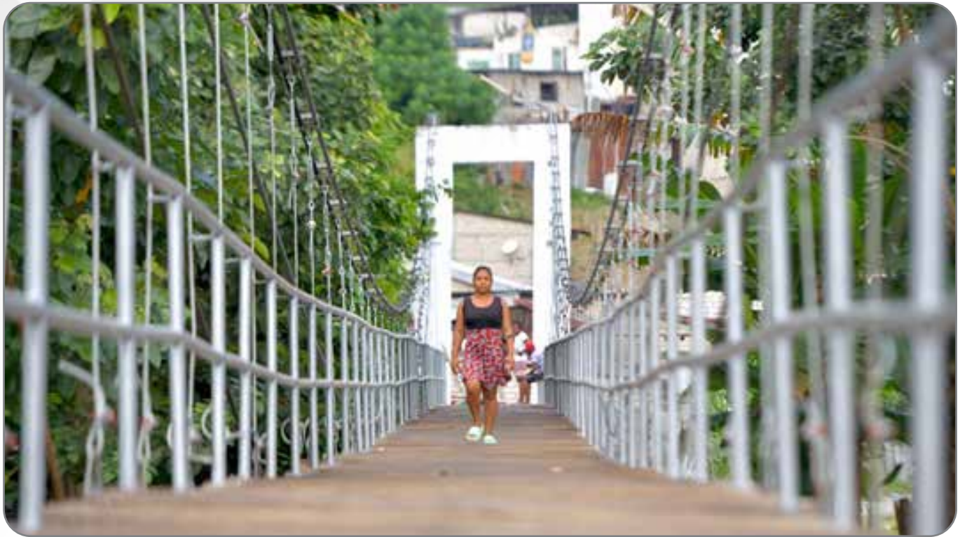
The rehabilitated pedestrian bridge benefits about 630 inhabitants of the island.
