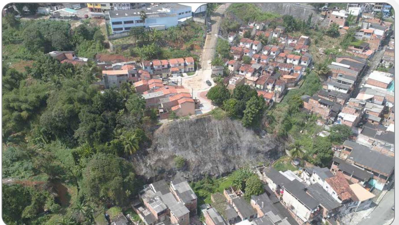
Slope Containment and Slum Urbanization at PDE 124
