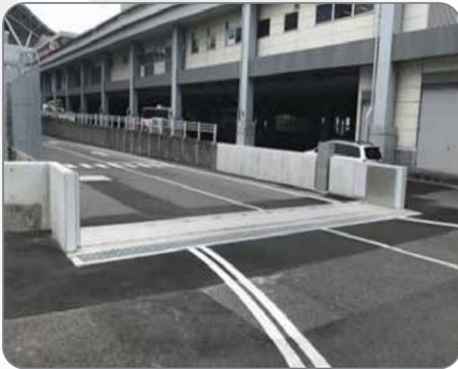
Flood counter-measures being implemented at Kansai International Airport
