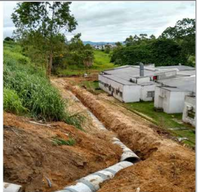
Drainage System at Santa Vitoria Community
