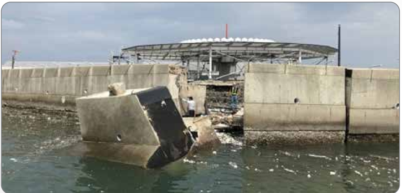
Disaster countermeasures being installed at Kansai International Airport after typhoon on 4th September, 2018
