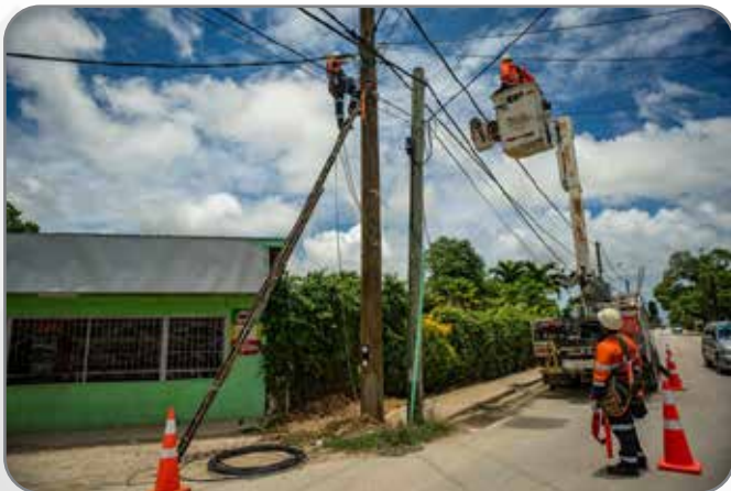
Maintenance activities of energy infrastructure in Tonga
