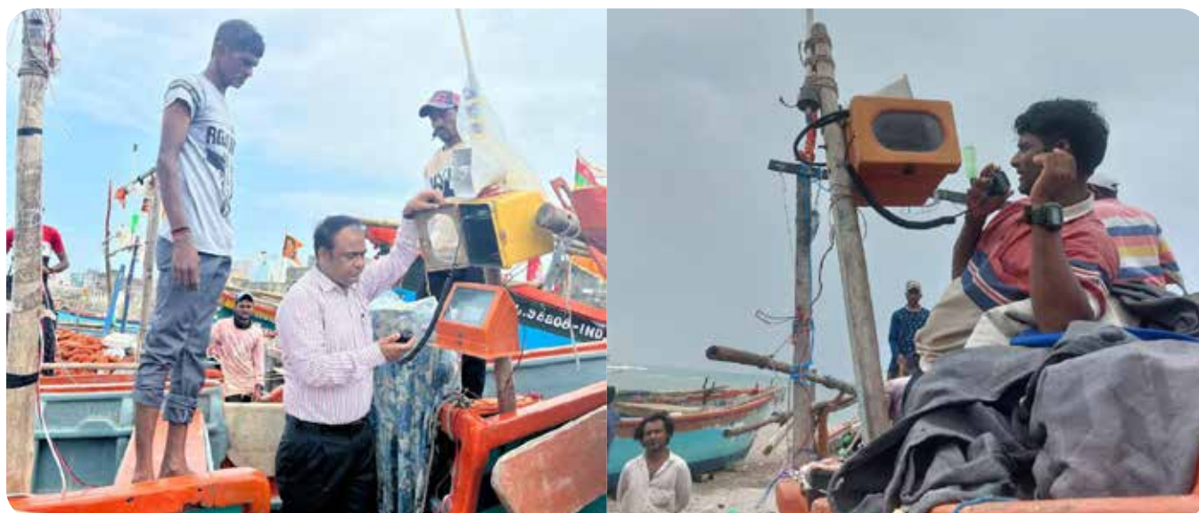
Coastal Telecom Resilience Field Test, Gujarat, Inde
