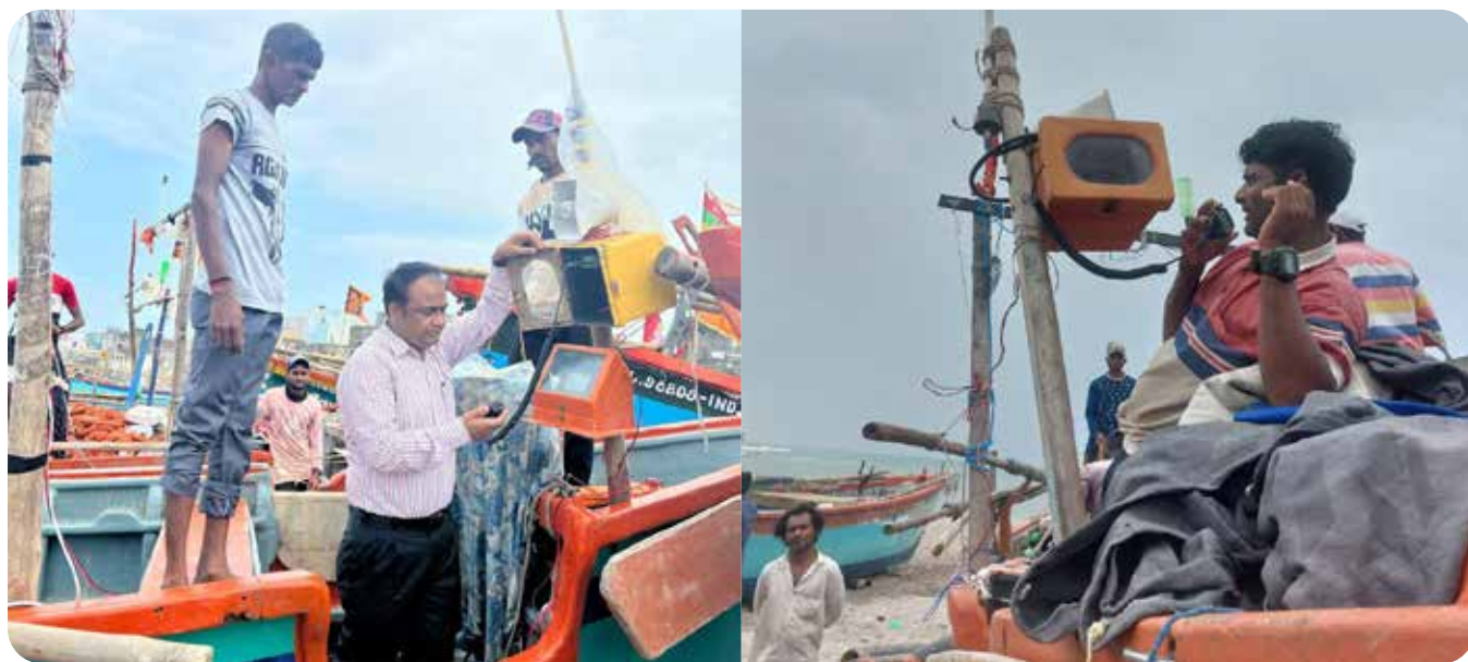
Coastal Telecom Resilience Field Test, Gujarat, India
