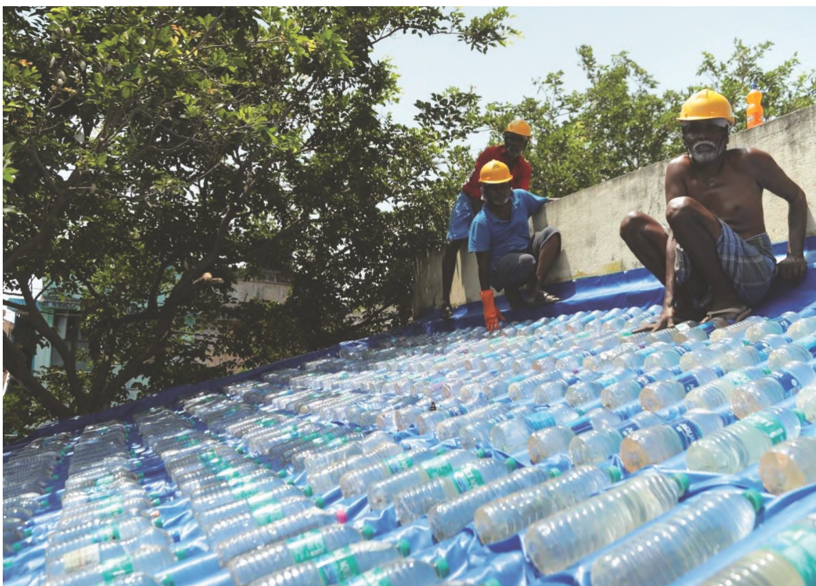
Installation of PET Bottles on the roof of a community centre in Chennai, India.
