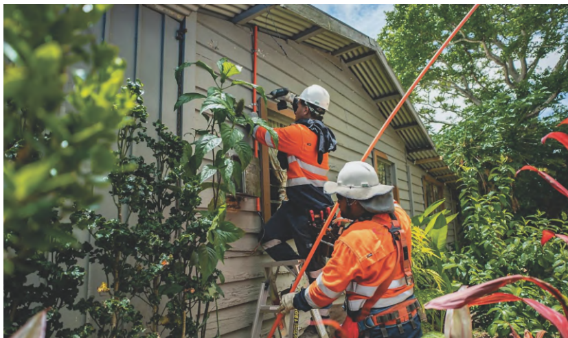
Installation of electric conduits on building walls Source: Asian Development Bank
