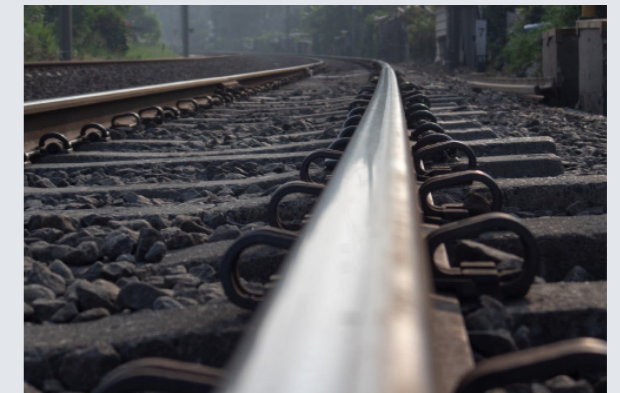
Image 4.2: White-painted train rails can remain 5-10°C cooler, helping to reduce heat expansion and the risk of buckling
