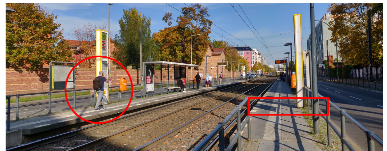
Image 3.1: A tram stop at the entrance of a major urban hospital features narrow platforms, creating challenges for wheelchair users and caregivers to access the stop and wait safely
