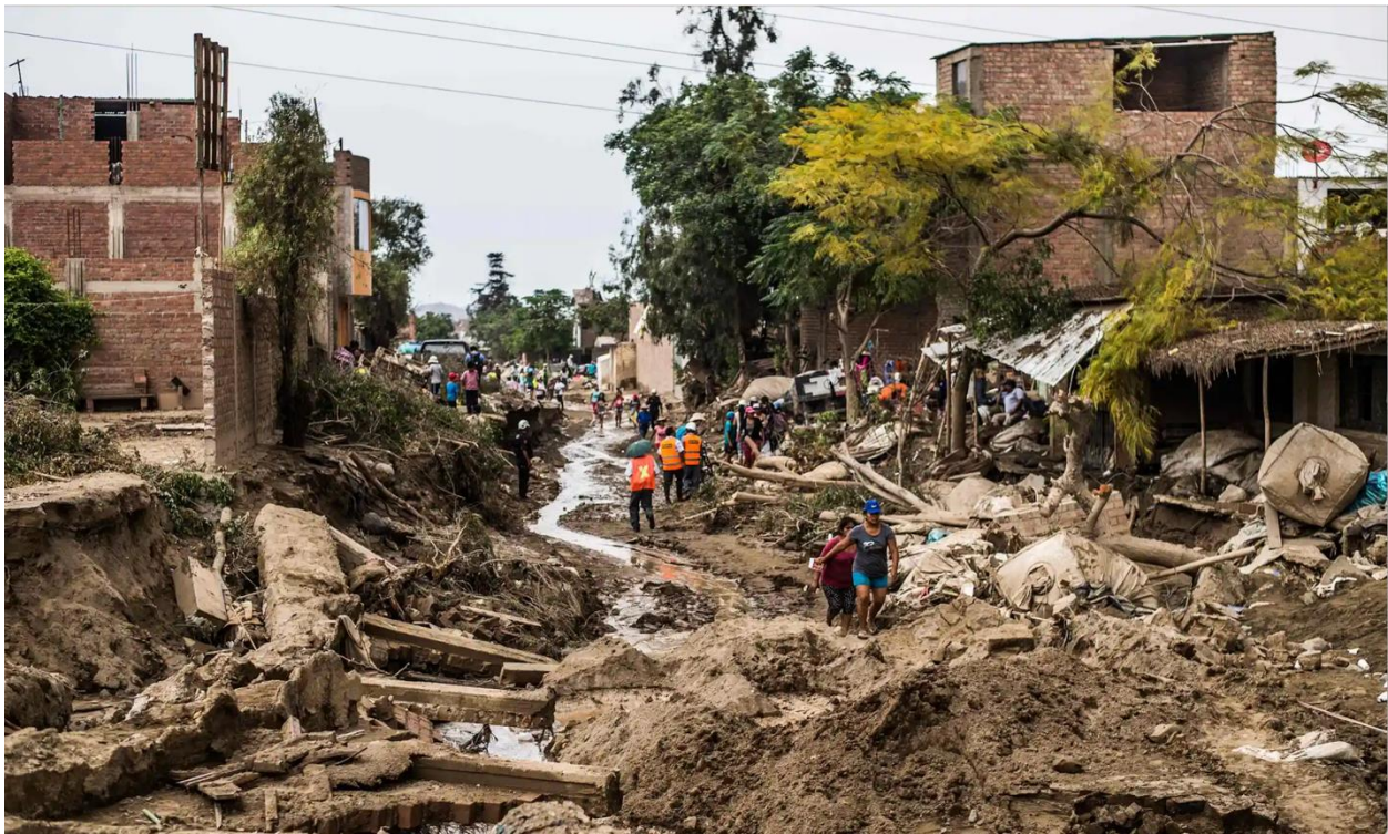
Figure 2: Gully erosion and loss of infrastructure from a powerful El Niño rainfall event, Lima, Peru 2022
