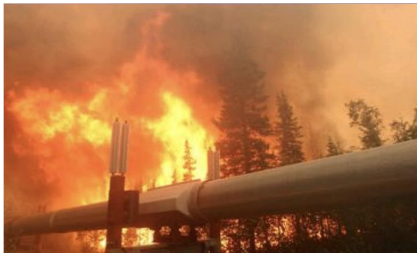
Figure 16: Oil pipelines throughout the arctic are subject to cracks and breaks as piling is undermined by permafrost melting and impacts from wildfire resulting from drying surface vegetation. Photo credit Michael Coffey, Alaska Department of Transportation
