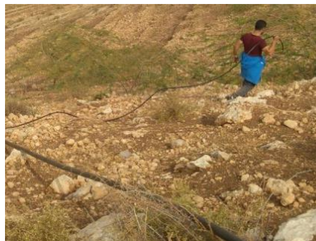
Installation of an Irrigation system in Jerash Governorate
