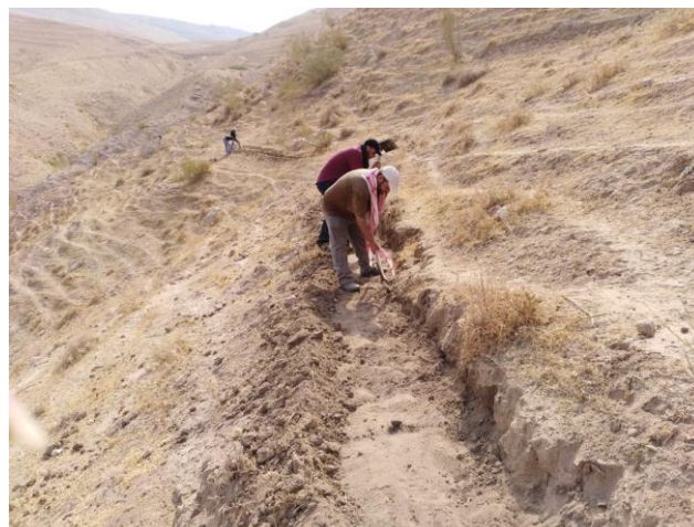
Terraces building in Albalqa governorate
