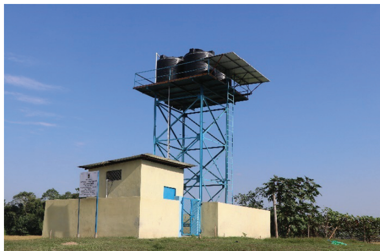
Figure 43. Village water facility
