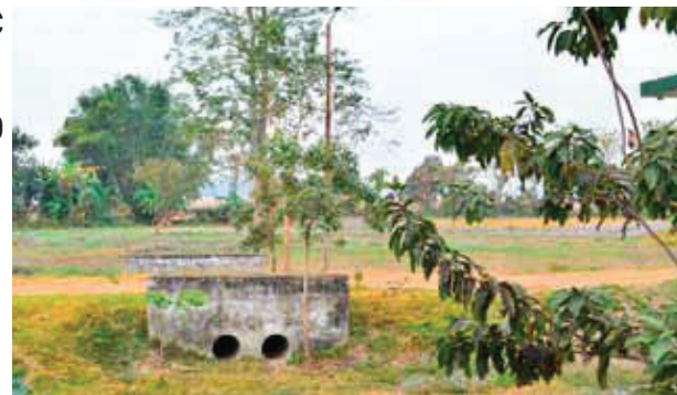
Figure 21. Road as embankment
