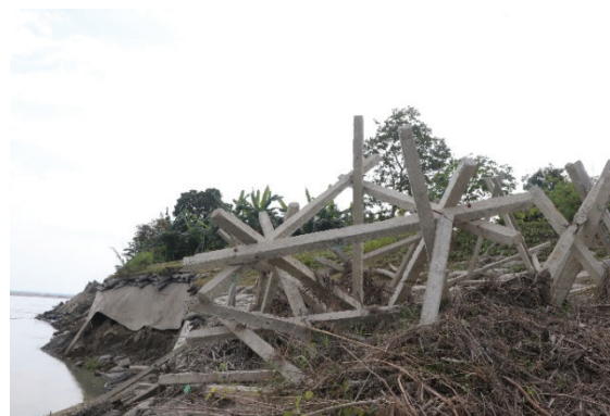
Figure 15. (b) RCC porcupines
