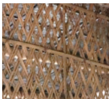
Figure 40. Ventilation jali pattern
