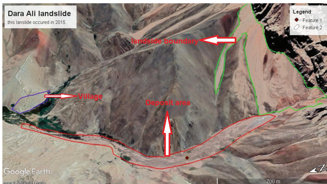
Figure 7. Google Earth photo of Dara Ali, Yakawalang landslide
