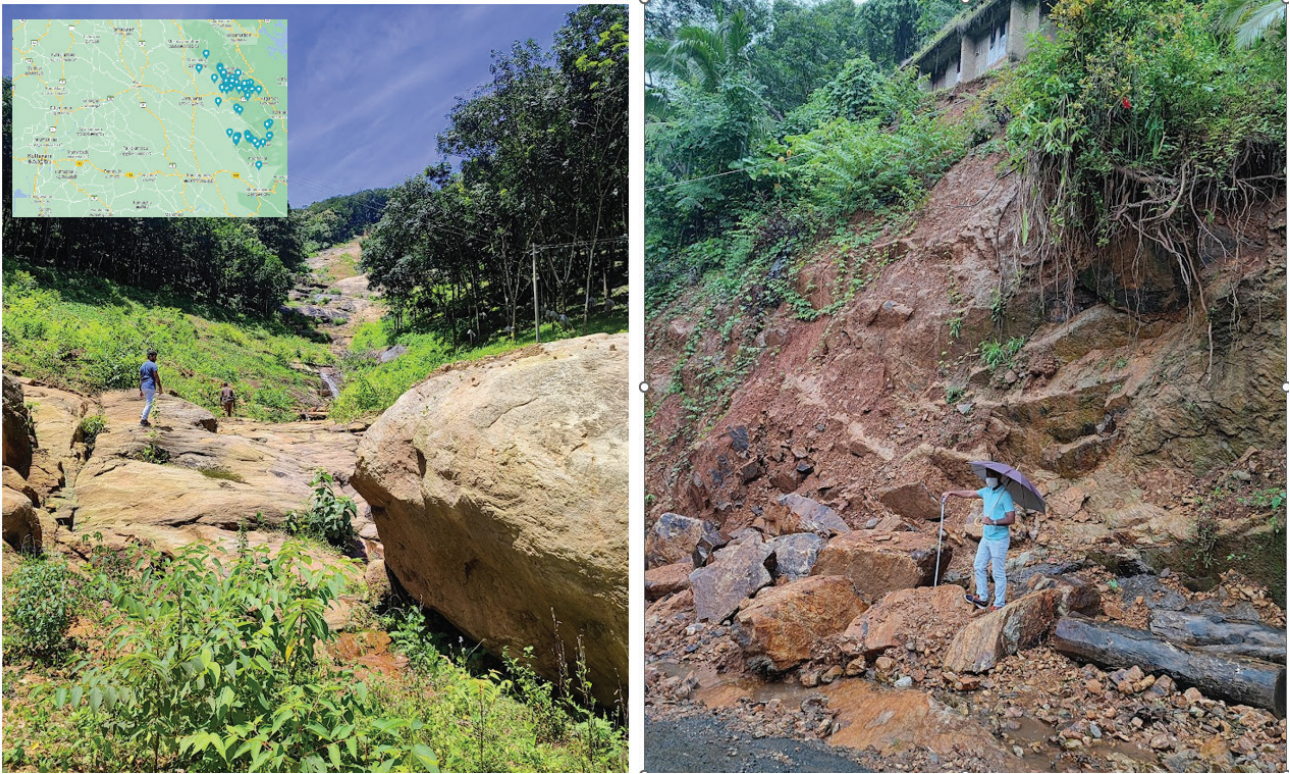
Figure 20. Site photos from field survey at Kottayam
