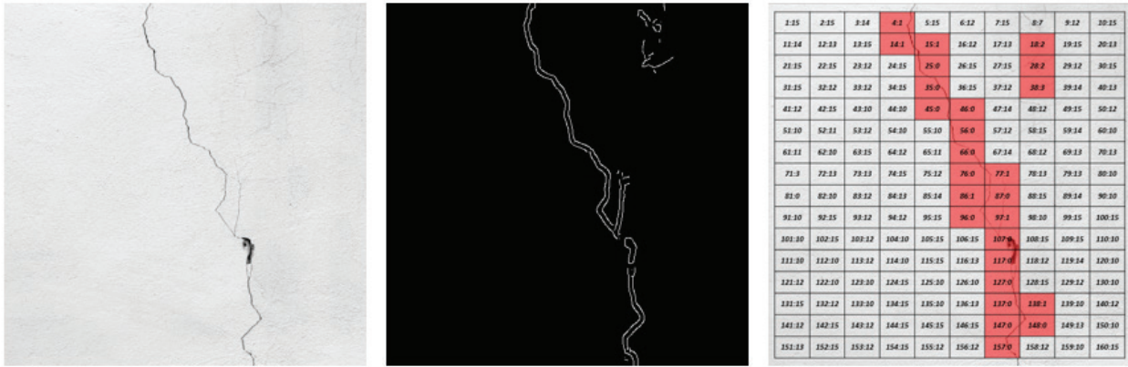
Figure 12. Cracks Categorization Matrix Distinguish Crack Pixels Based on Pixel Width
