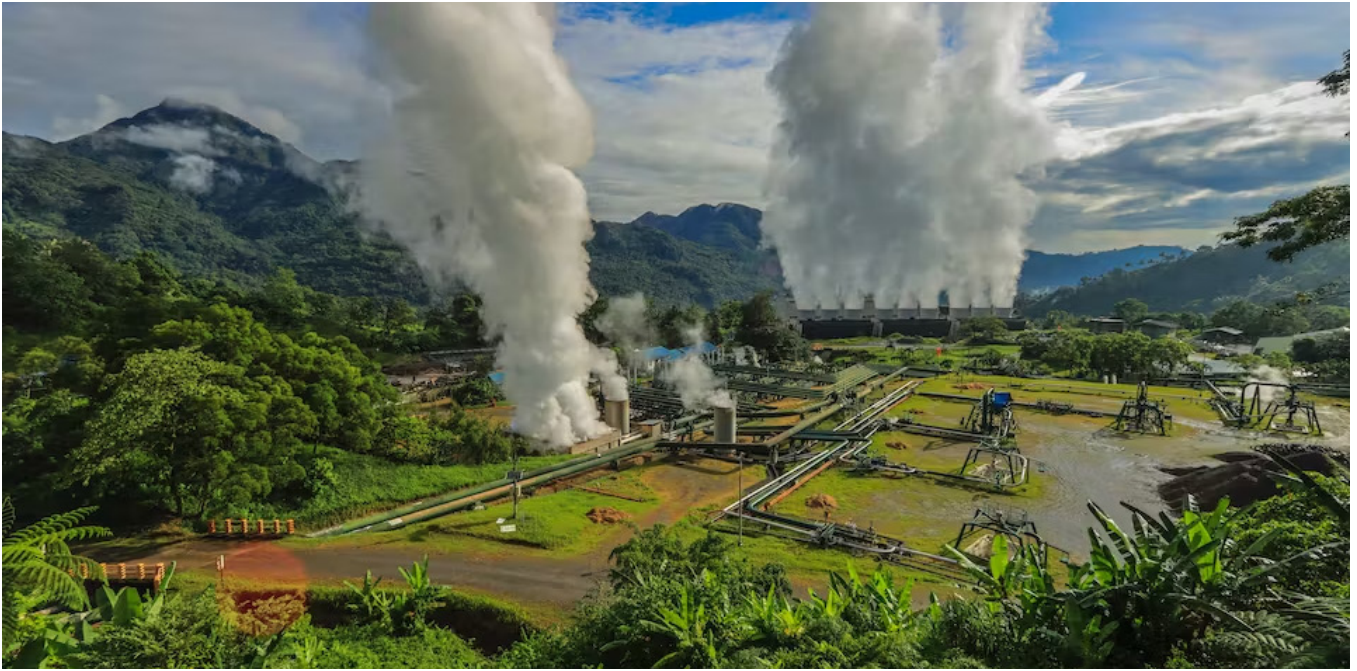
Geothermal Power Plant, Philippines. Source: EDC
